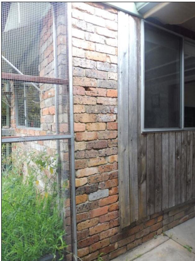
Figure 5.11 The rear wing has been extended and modified and has varying brick and lightweight walls and infill and aluminium framed windows. The brick and later infill indicates at least two additions.
