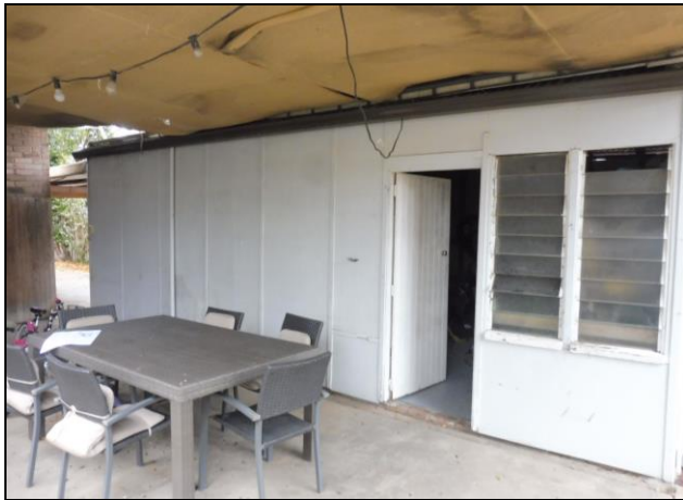
Figure 5.13 The garage is constructed on a concrete slab and is a simple timber framed structure clad in FC sheeting with gabled roof clad in metal sheeting.
