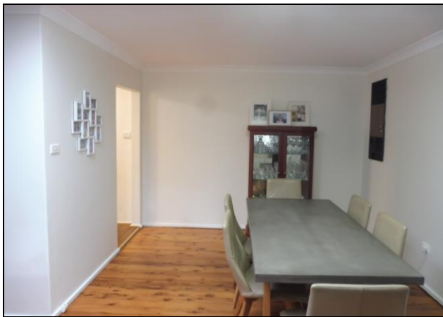
Figure 5.27 The original rear wing has been opened up, modified and extended and has a modern timber floor and plasterboard ceiling with simple coved cornice.
