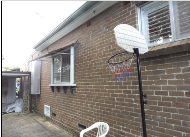
Figure 5.9 The western elevation. The window openings have generally been modified and windows have been replaced.
