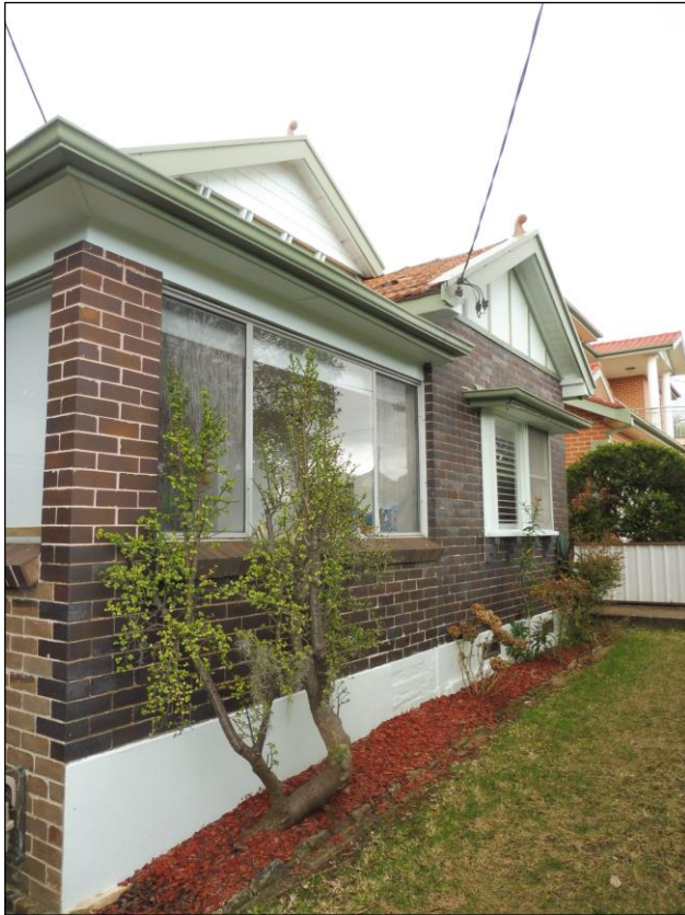
Figure 5.4 The front façade has timber windows, which appear to have been altered, and aluminium framed windows added later to infill the verandah which has a modified, flat roof clad in metal sheeting. Some infill is visible in rendered base and brickwork at the front and the brick post also appears to have been added.
