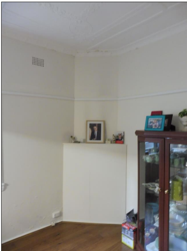
Figure 5.25 The hall leads into a dining room that retains a narrow splayed fireplace breast, however, the fireplace has been removed and sheeted over.
