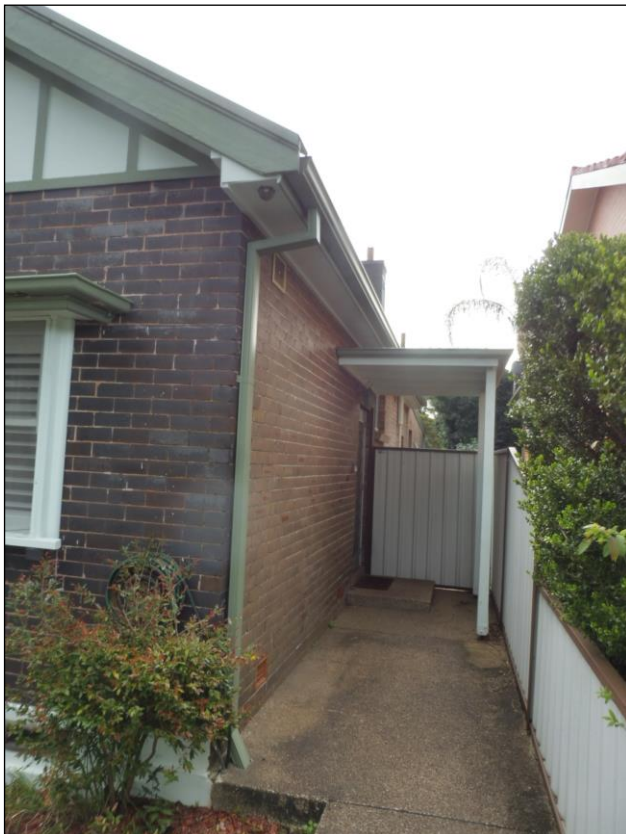
Figure 5.5 The eastern setback, pedestrian path and building entry. A timber framed, lightweight awning, fencing and step have been added.
