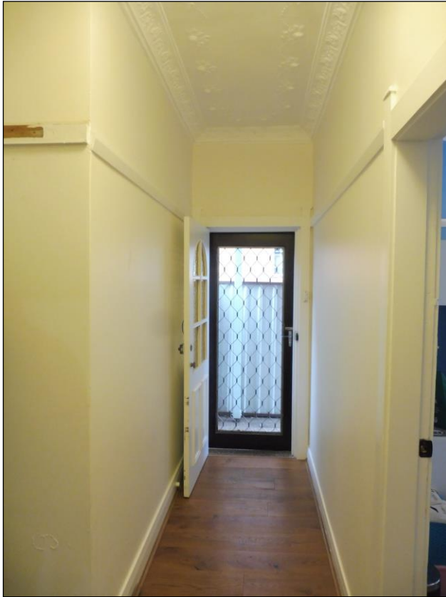
Figure 5.20 The interior has timber floors, high plaster and plasterboard ceilings and timber joinery. The main rooms and bathroom are located about and accessed by a kinked hall that extends from the side entry.
