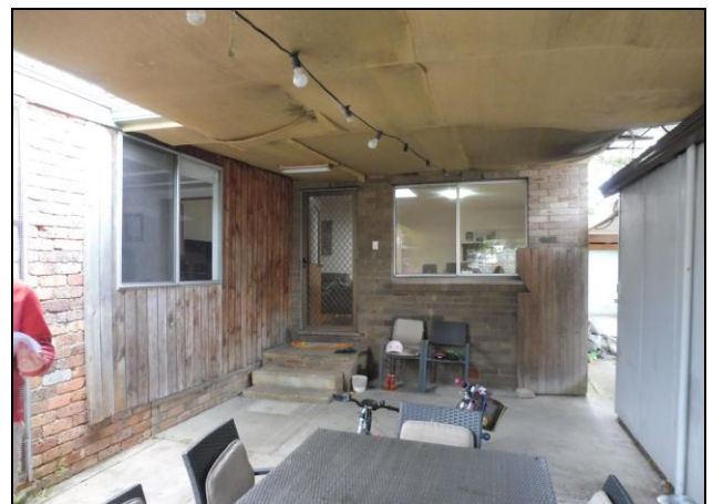
Figure 5.11 The rear wing has been extended and modified and has varying brick and lightweight walls and infill and aluminium framed windows. The brick and later infill indicates at least two additions.
