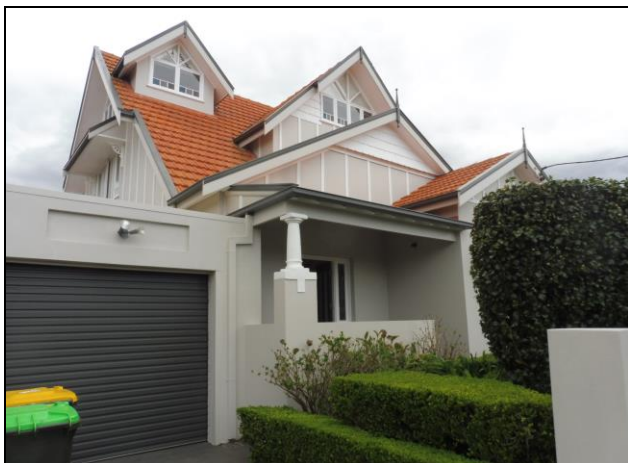
Figure 4.12 No. 7 has been rendered with upper level and attic added and accommodated within the steep pitched gabled roof. A garage has also been added in the western side setback.
