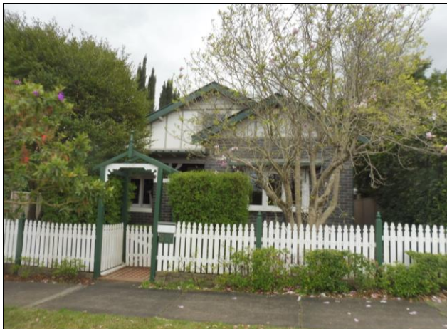
Figure 4.10 No. 5 Ayr Street is a single storey, face brick and bagged Inter-war dwelling. The house retains the two street facing gables and an open front verandah. A large addition that extends into the western side setback has been constructed at the rear.
